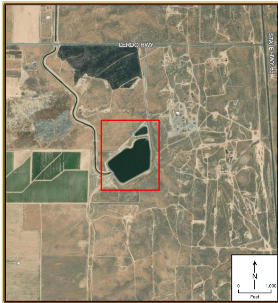
Figure 4. District Reservoir “B”
